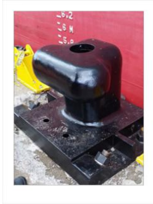
Mooring bollard perfectly installed at port
