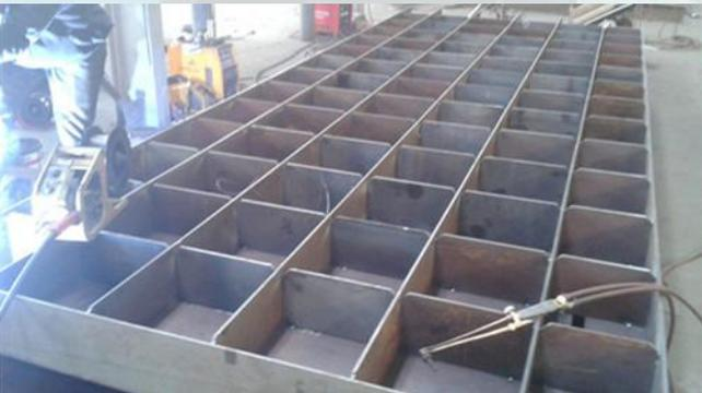
Locating and primary welding the cutting plate according the design drawings.
